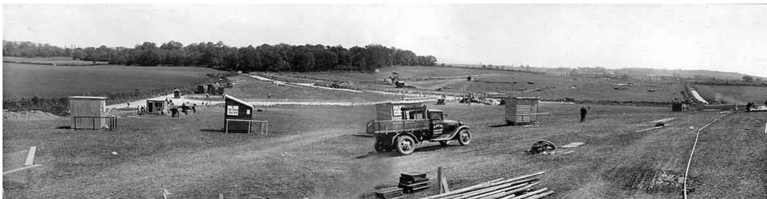
Start of construction May 1939
