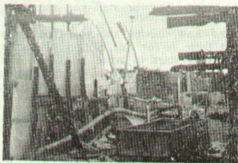
Charred remains of the Drying Room
