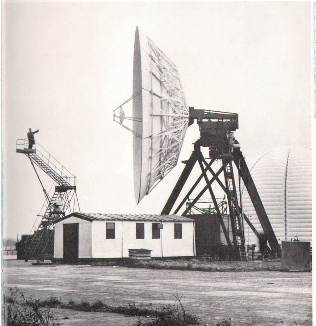
Royal Signals man one of the three air transportable satellite communications ground stations. These stations are taking part in a joint project with American military authorities using a series of near-synchronous satellites launched by America and which started in the spring of 1966. The photograph shows the 40-ft. diameter dish aerial eventually to be installed inside the 60-ft.-high inflatable radome seen in the background.
