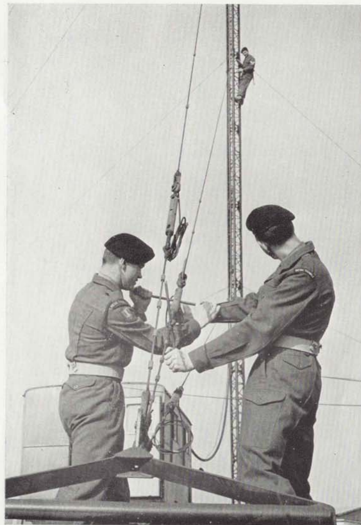
Erecting a Radio Mast in Germany.
