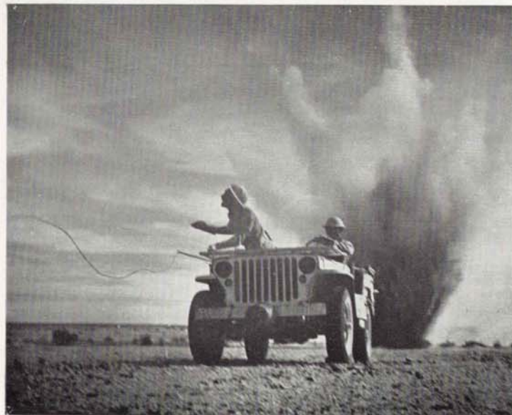
Laying cable while under fire in the Western Desert—1942.
