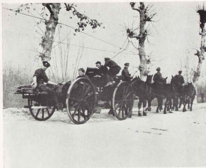
A Cable Wagon used for laying lines during the First World War.
