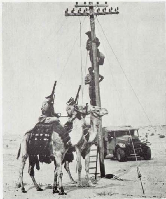
Sinai Desert, 1943. Linemen repair a fault in what was the longest Military Trunk System in the world—5,000 miles from Algiers to Teheran and built by Royal Signals.
