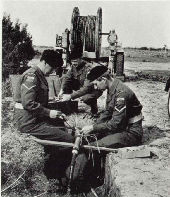
Cable Jointers lay underground cable in Cyprus.
