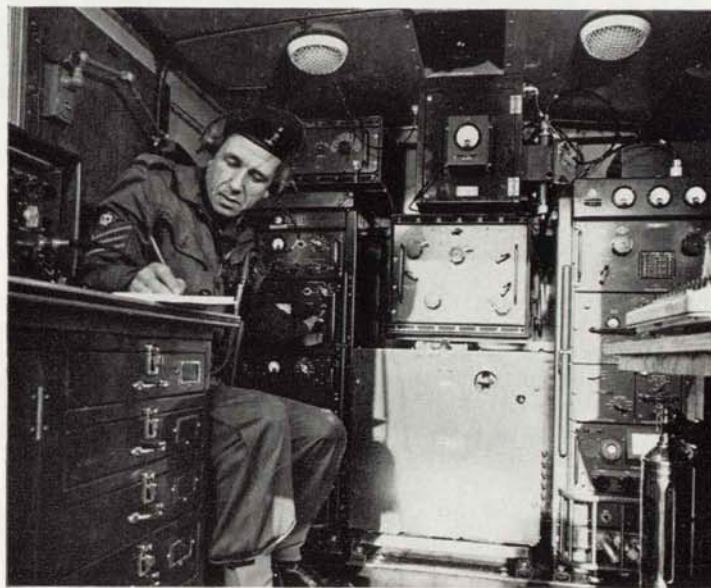
A Yeoman of Signals formerly a Telegraph Operator receiving morse on a Radio Station D11/R230 which has a range of over 1000 miles.
